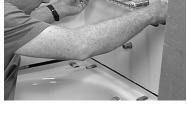
Measure the distance from the top of a shim on the tub ledge to the center of each pipe. See Figure 17.6.4.D.
