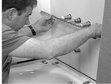
Measure the distance from the top of a shim on the tub ledge to the center of each pipe. See Figure 17.6.4.D.
